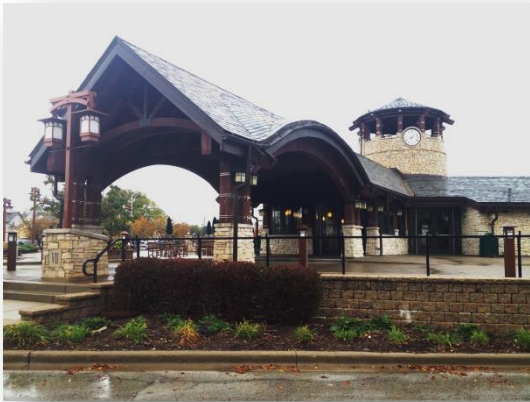
Tinley Park Metra Station. Photo Credit: RTA
